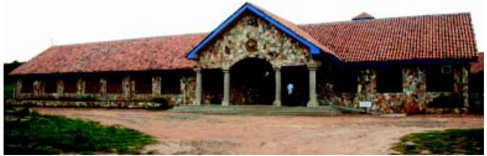
New Administration and Library Building at Ghana Christian University
